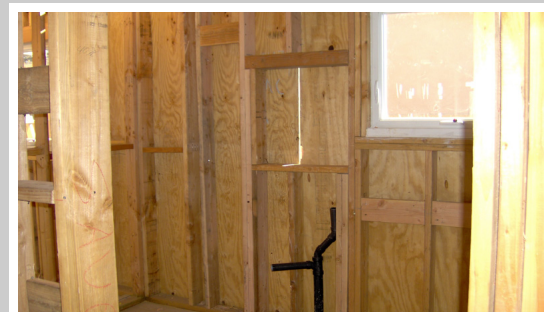
Dec 20, 2005 — Plumbing started.
