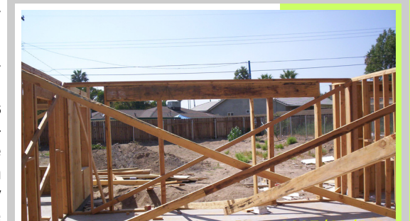
Sep 01, 2005 — Framing started.
