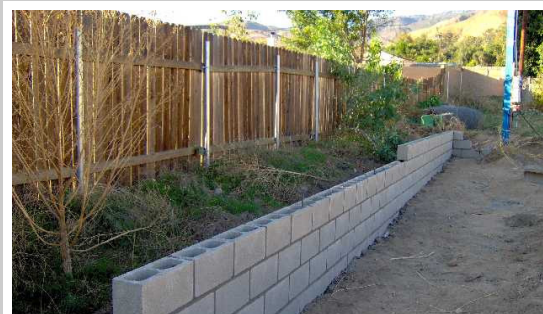
Oct 27, 2006 — Perimeter walls started
