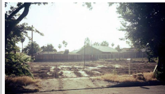
June 2005 — Final grading.
