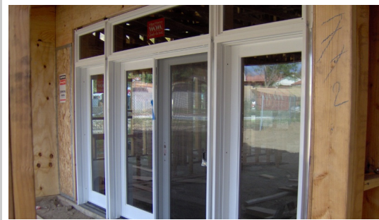
Nov 06, 2005 — Back door installed.
