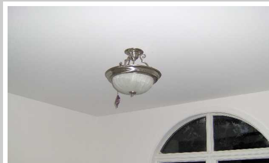
Oct 04, 2006 — Finish Electrical
